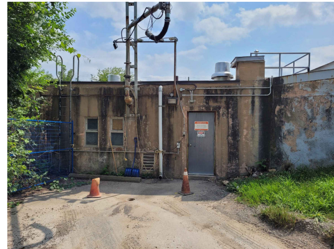
PHOTO No. 1 - EXTERIOR CLADDING ON DIGESTER BUILDING N.T.S.
