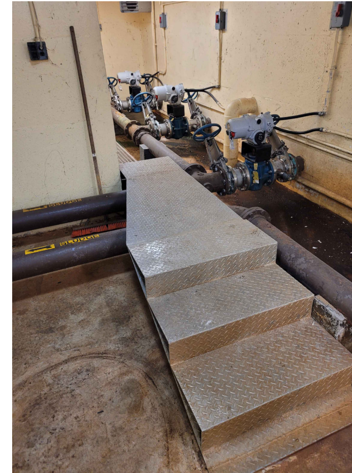
PHOTO No. 1 - ALUMINUM CHECKER PLATE RAMP (TUNNEL) N.T.S.
