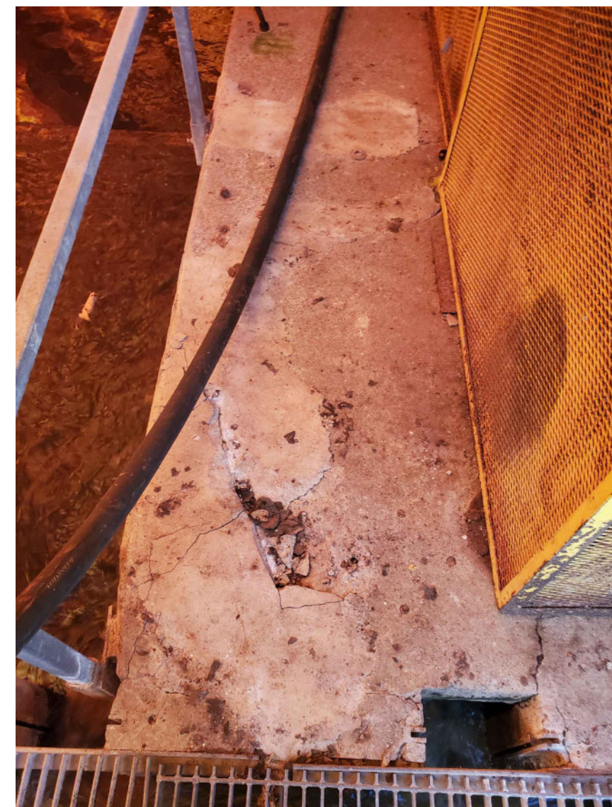
PHOTO No. 1 - TYPICAL HORIZONTAL CONCRETE REPAIR N.T.S.
