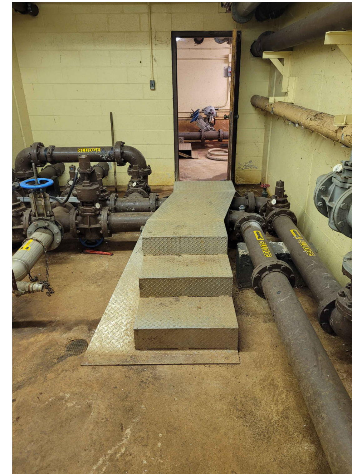
PHOTO No. 2 - ALUMINUM CHECKER PLATE RAMP (CONTROL BUILDING BASEMENT) N.T.S.
