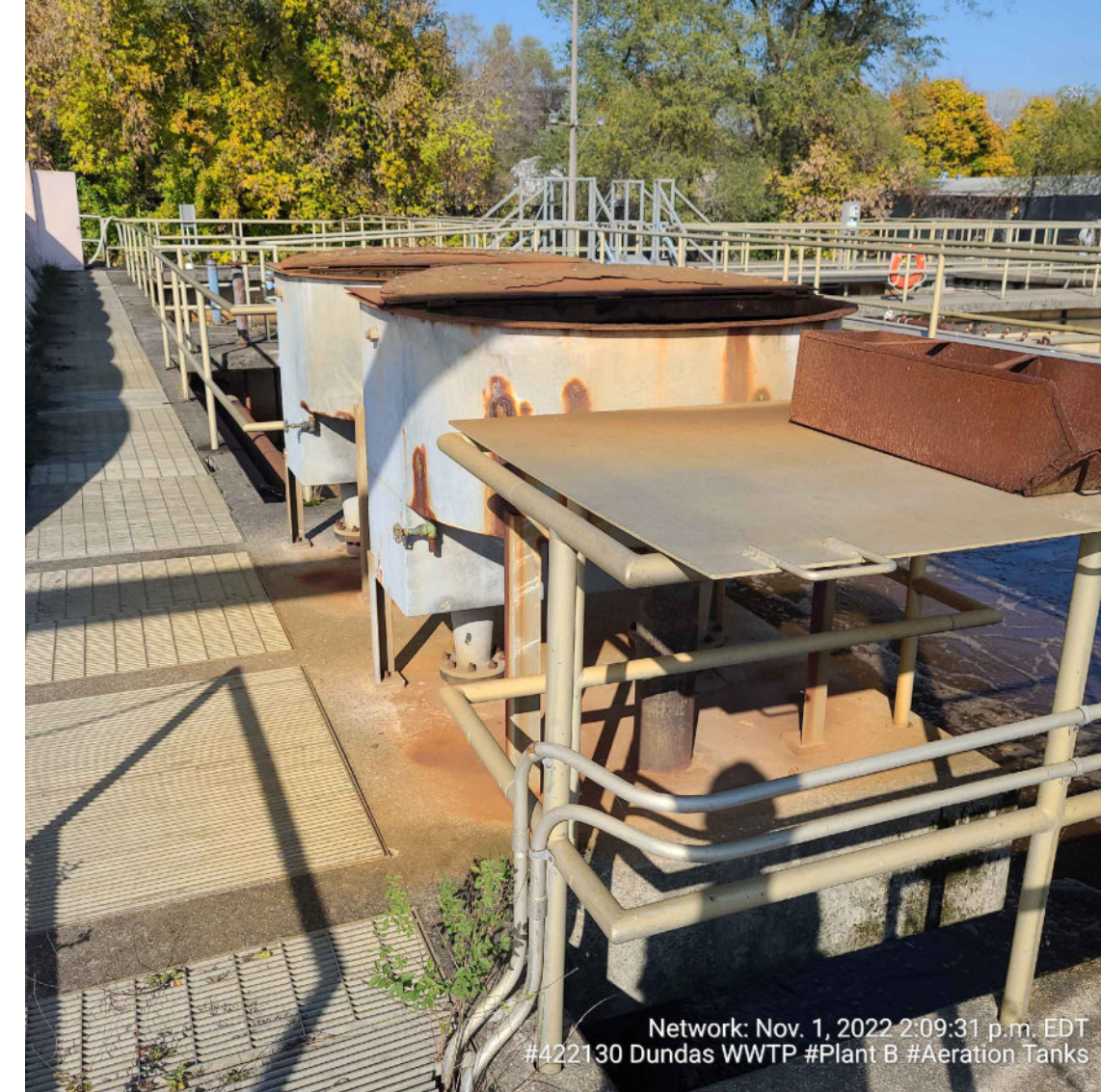
PHOTO No. 1 - EXISTING SPLITTER BOXES N.T.S.
