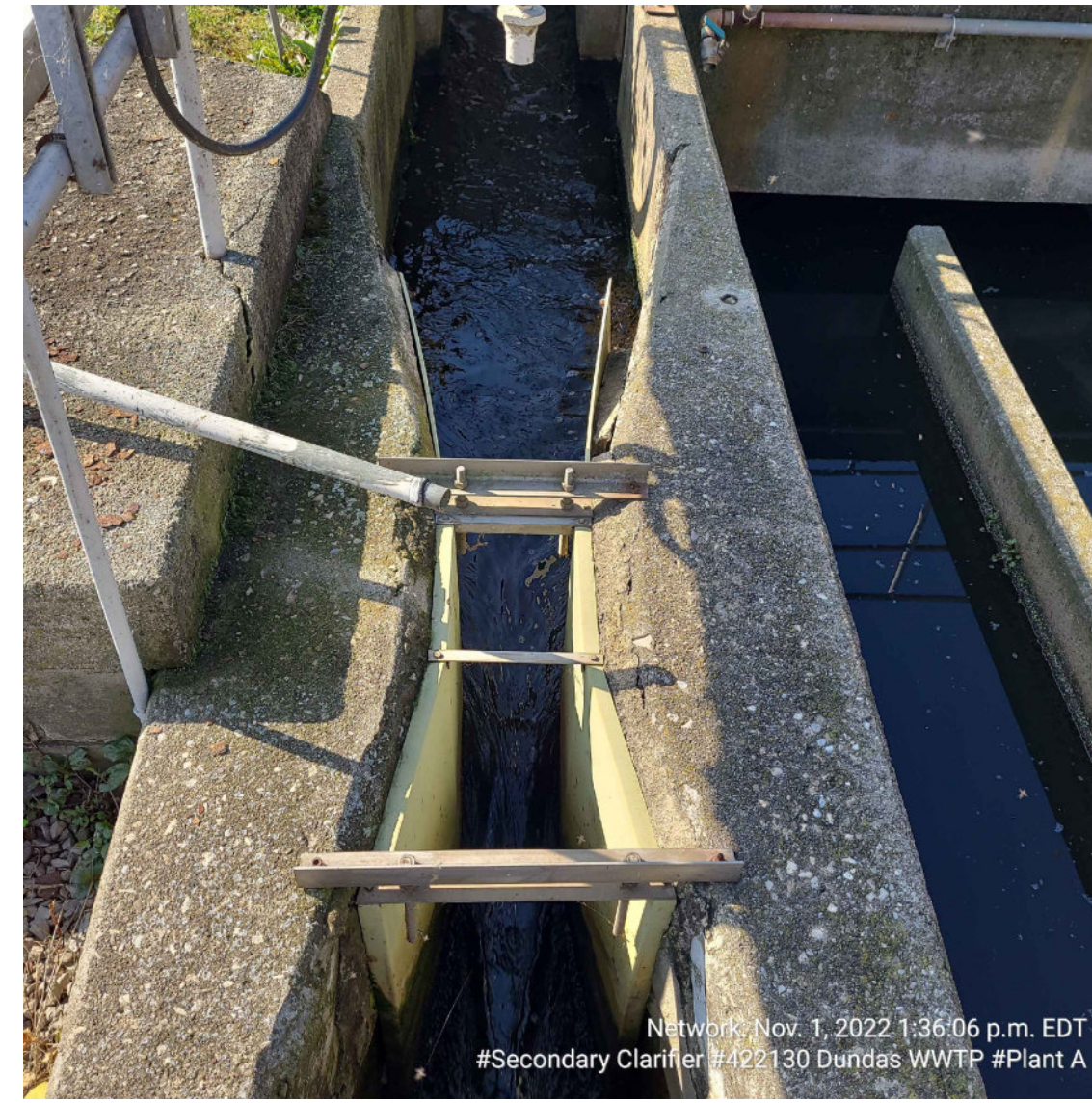
PHOTO No. 1 - PLANT A PARSHALL FLUME N.T.S.
