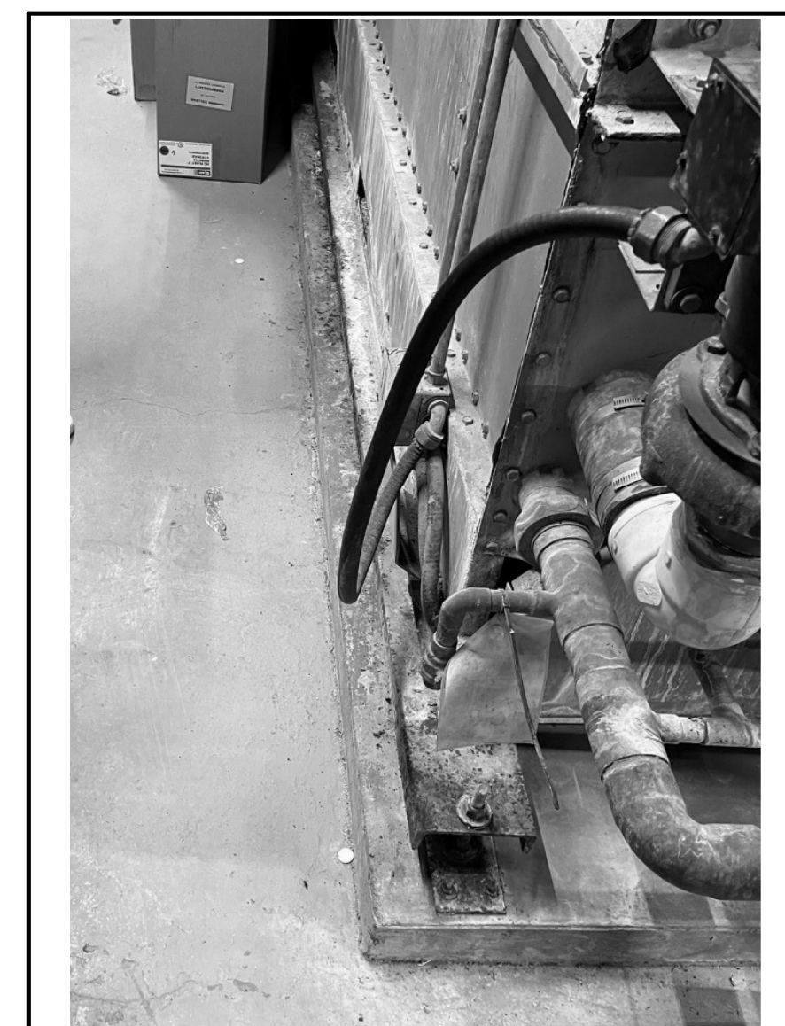
8 EXISTING COOLING TOWER DRAIN PIPING ME101 N.T.S.
