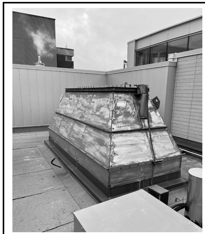
4 EXISTING COOLING TOWER DISCHARGE HOOD ME100 N.T.S.
