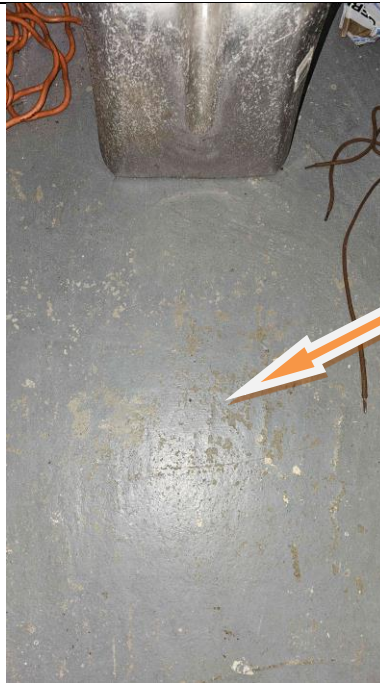
Photo 4 – Lead-containing grey paint on basement floor.
