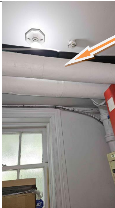
Photo 2 – Asbestos-containing aircell insulation on pipe straights.
