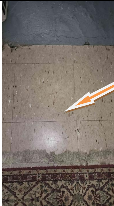
Photo 3 – Non-asbestos 12" x 12" beige with brown and white flecks vinyl floor tile and mastic adhesive (VFT-01).
