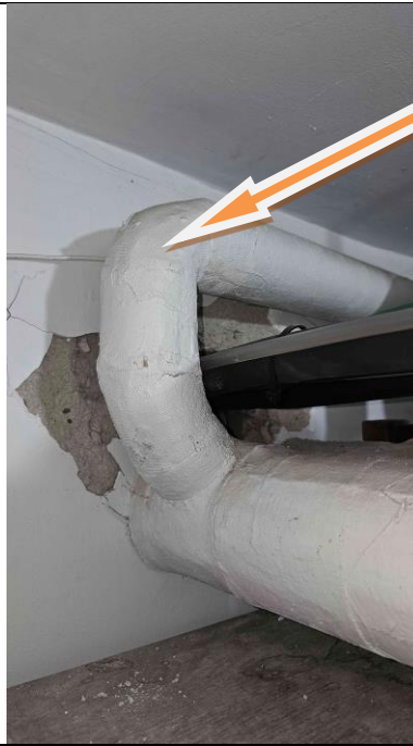
Photo 1 – Asbestos-containing paring cement on pipe fittings.
