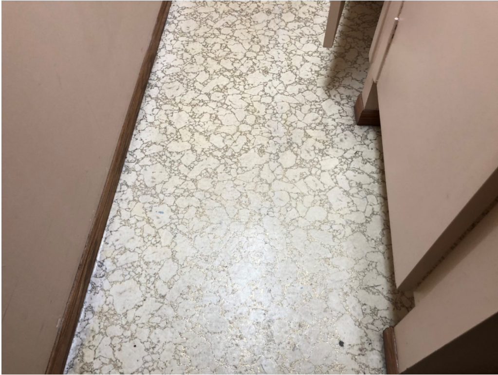
Photograph No. 3 – Vinyl sheet flooring within the foyer washrooms is asbestos-containing.
