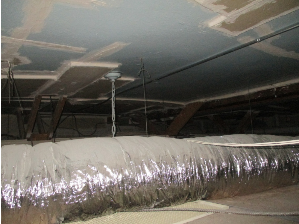
Photograph No. 1 – The skim coat layer of plaster walls and ceilings throughout the Site is considered asbestos-containing.
