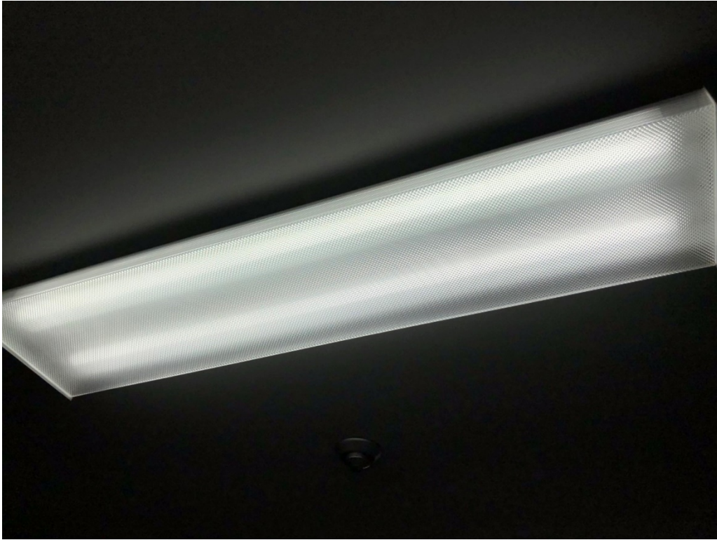
Photograph No. 7 – Fluorescent light tubes are suspected of containing mercury, and florescent light ballasts are suspected of containing PCBs.
