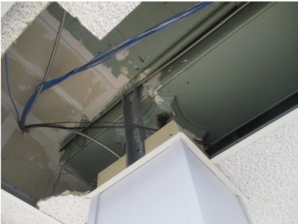
Photograph No. 2 – Green paint above ceiling tiles in the Basement area is lead-containing.
