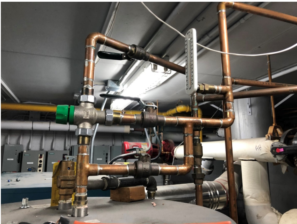
Photograph No. 6 – Solder joints on copper pipes are suspected of containing lead.
