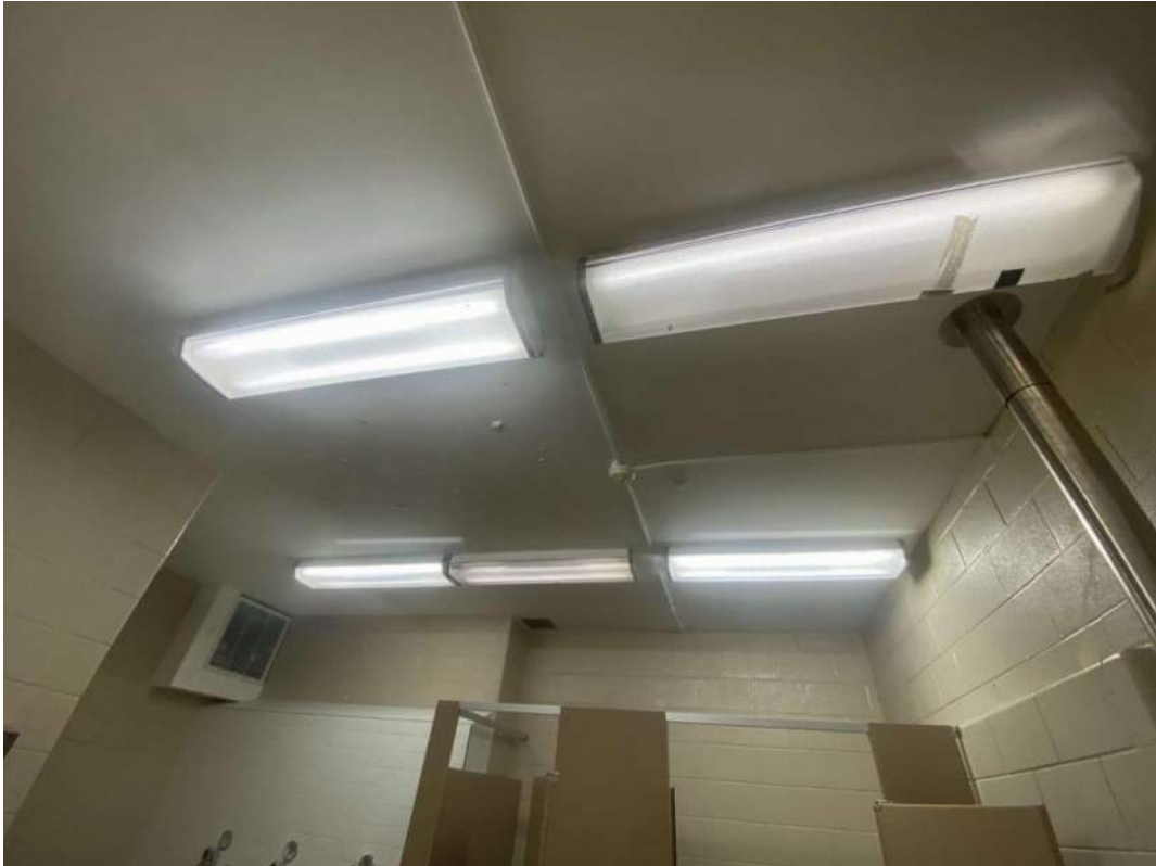
S0003A (None), Ceiling, Drywall and joint compound, Boy's Washroom (Location #: 9212)
