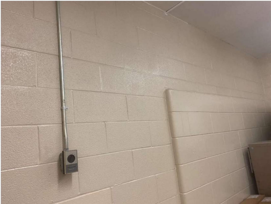
S0018C (None), South wall, Wall, Paint, Boy's Washroom Storage (Location #: 9213)
