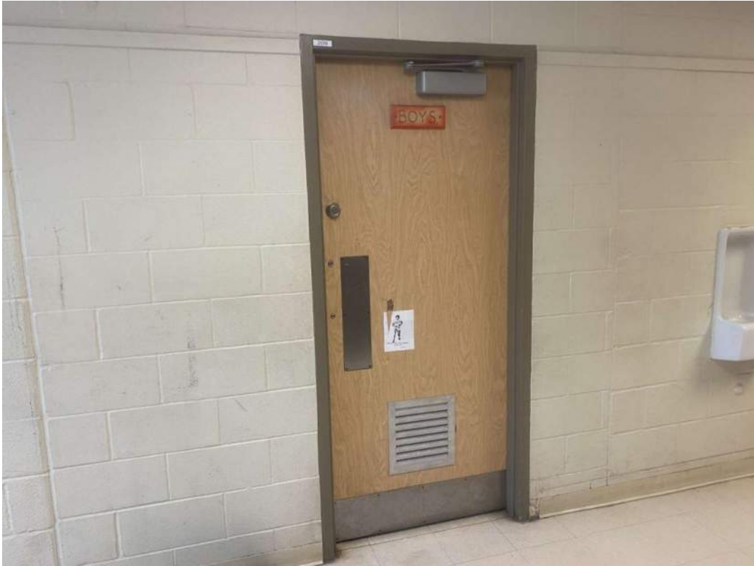
S0025A (None), Outside boys washroom, Wall, Paint, Corridor (Location #: 9264)
