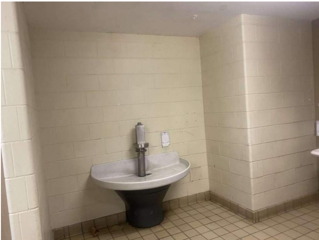
S0024B (None), South wall, Wall, Paint, Boy's Washroom (Location #: 9255)
