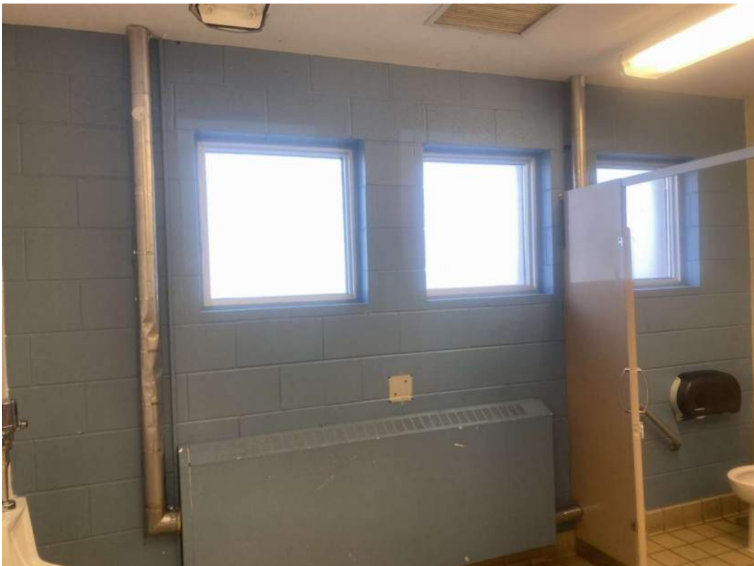
S0020A (None), East wall, Wall, Paint, Boy's Washroom (Location #: 9161)
