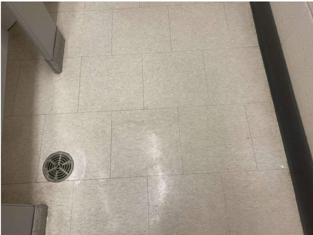
S0012A (None), 12x12 beige with brown and white fleck, Floor, Vinyl Floor Tile and Mastic, Male Staff Washroom (Location #: 9208)
