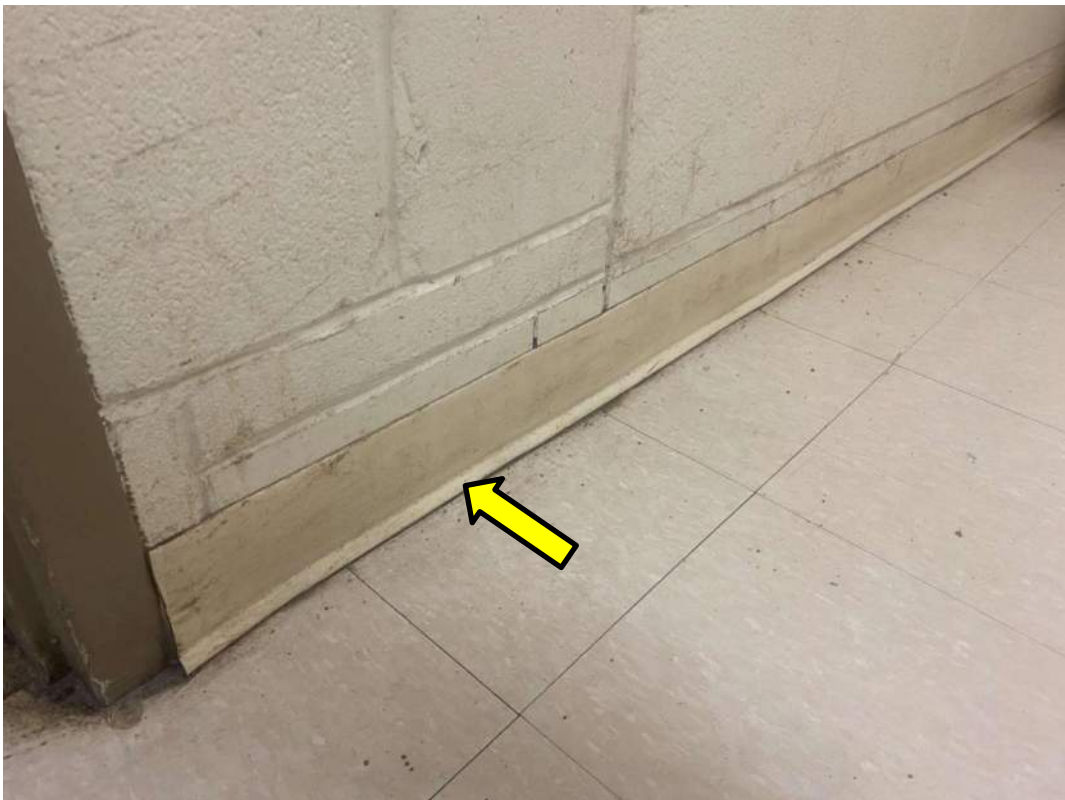
S0010A (None), cream baseboard, Wall, Mastic, Corridor (Location #: 9264)
