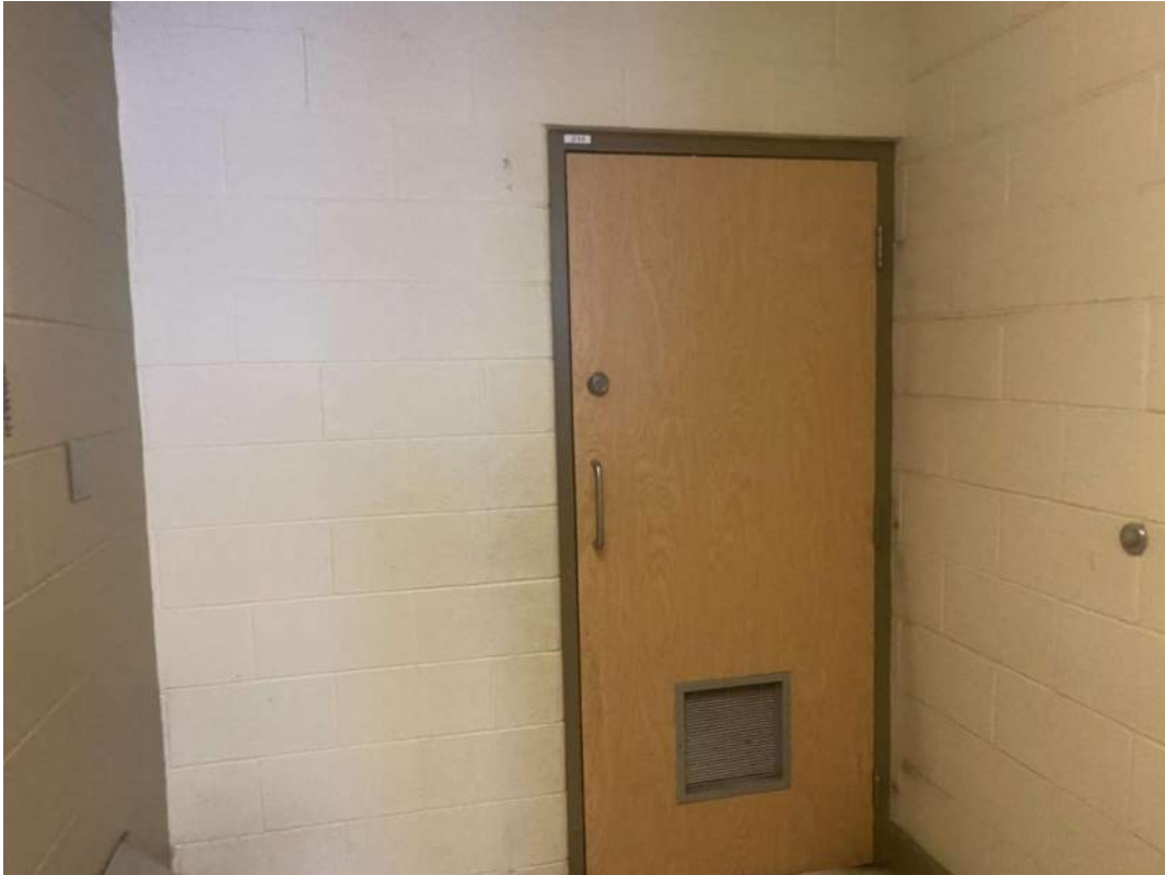
S0023C (None), West wall, Wall, Paint, Girl's Washroom (Location #: 9253)
