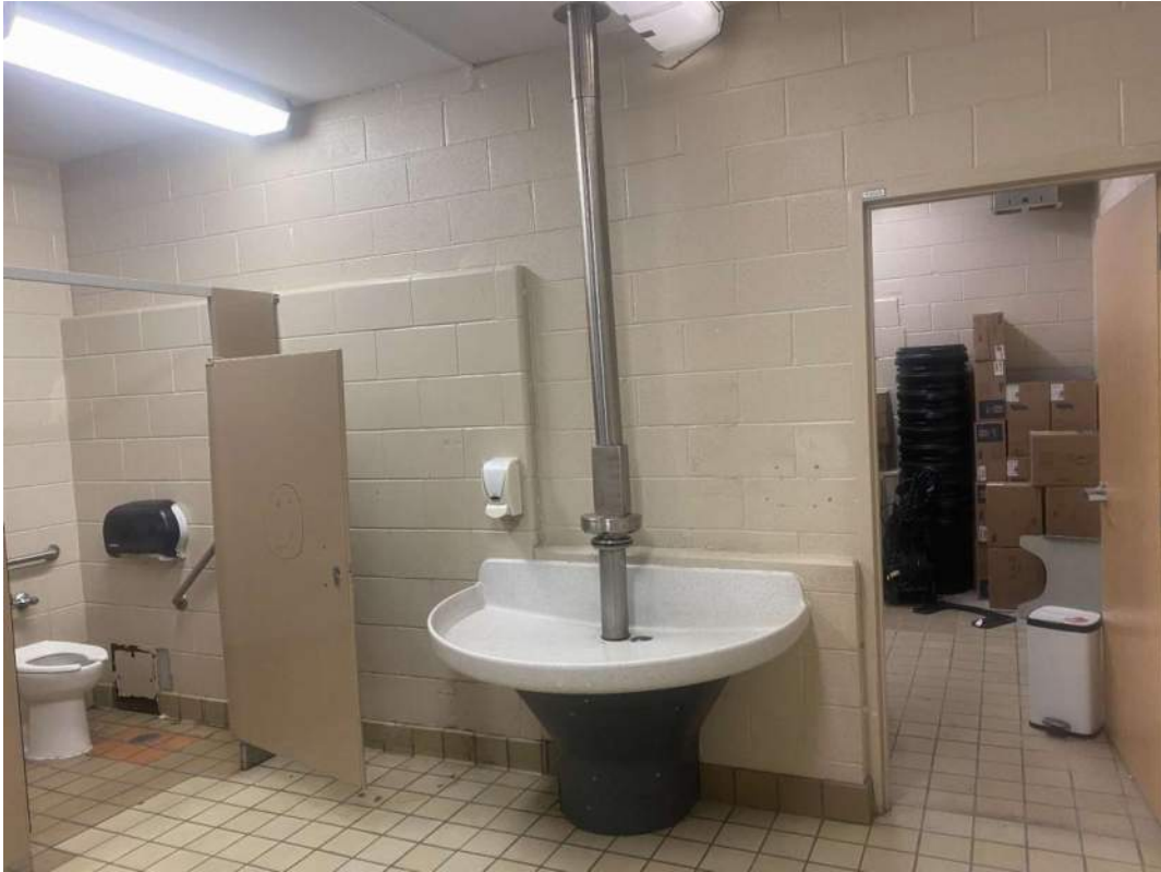
S0017A (None), North Wall, Wall, Paint, Boy's Washroom (Location #: 9212)
