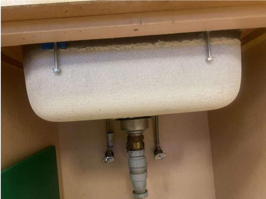
S0005A (None), white, Other, Sink, Mastic, Staff Room (Location #: 9206)
