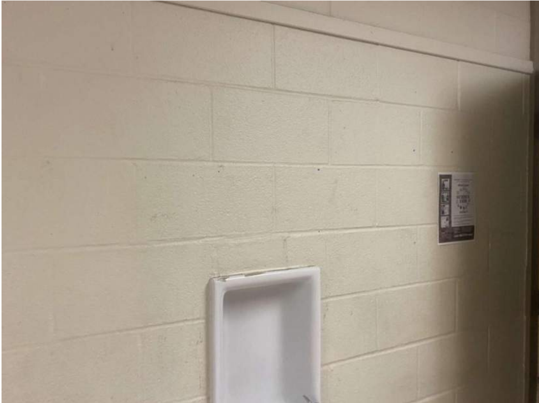
L0005(Lead, None), beige, Wall, Corridor (Location #: 9264)
