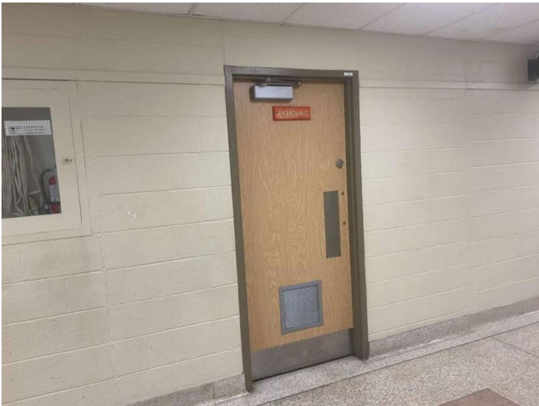
S0022B (None), outside girl's washroom, Wall, Paint, Corridor (Location #: 9183)
