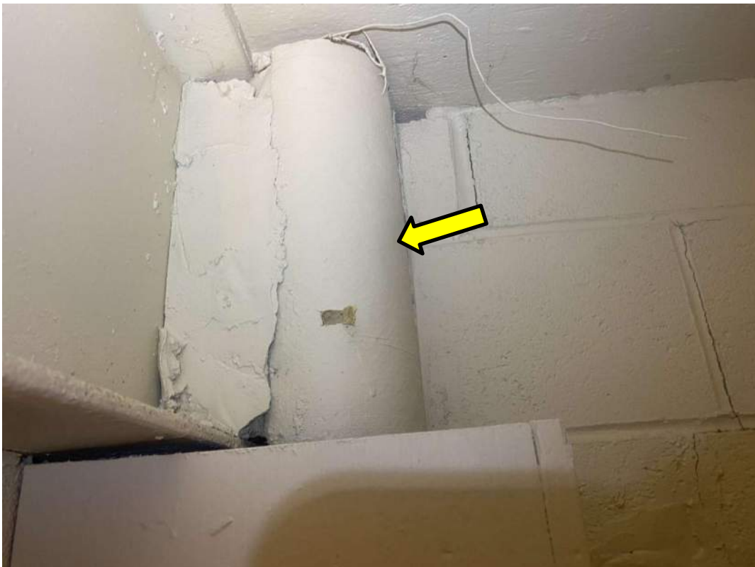
S0008A (None), Piping, Sweatwrap, Caretaker Area (Location #: 9162)
