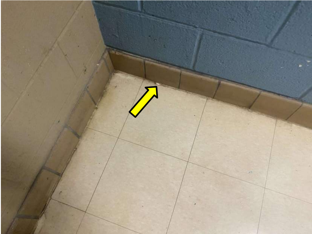
S0011A (None), white, Floor, Caulking, Boy's Washroom (Location #: 9255)
