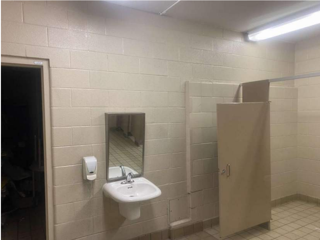
S0015A (None), North Wall, Wall, Paint, Girl's Washroom (Location #: 9210)
