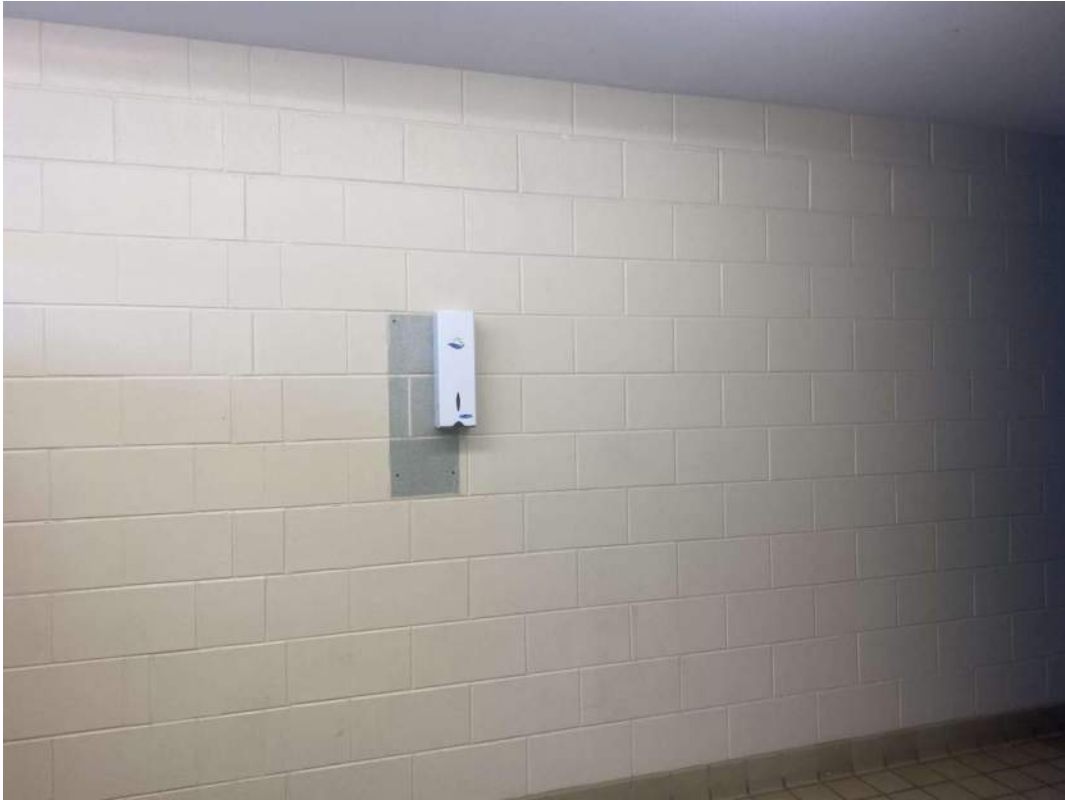
S0021B (None), South wall, Wall, Paint, Girl's Washroom (Location #: 9163)
