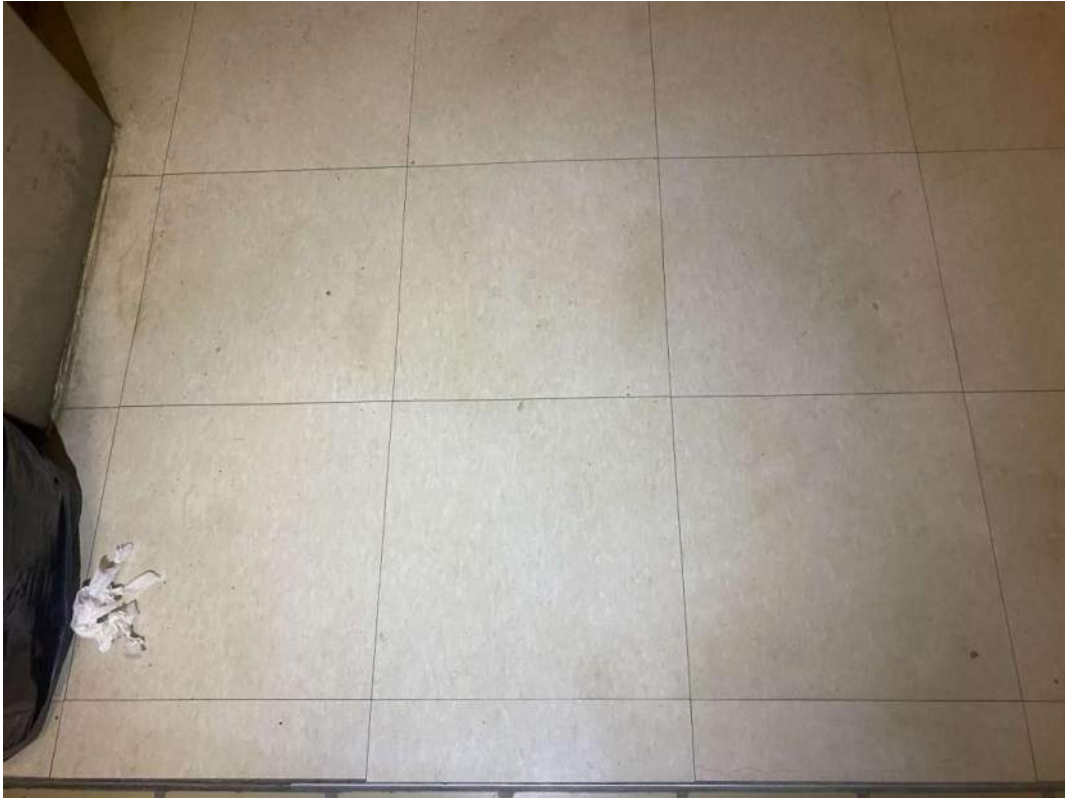
S0009C (None), 12x12 beige with white fleck, Floor, Vinyl Floor Tile and Mastic, Girl's Washroom (Location #: 9253)
