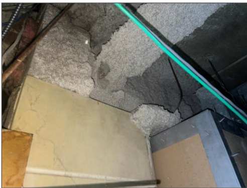
Non-asbestos grey fireproofing S0057A-C, Hallway (Loc. 1011)
