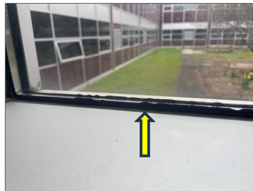
Non-asbestos black window putty, S0055A-C, Hallway (Loc. 1011)
