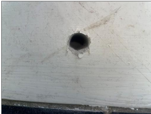
Vermiculite investigation hole, no vermiculite found.
