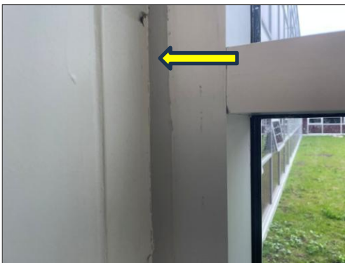
Non-asbestos grey caulking, S0052A-C, Hallway (Loc. 1011)
