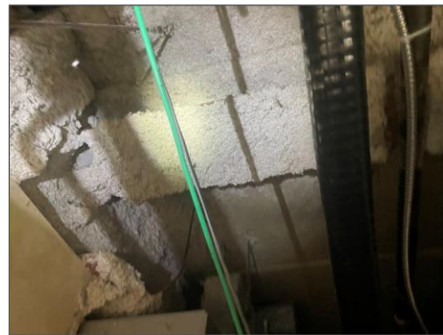
Non-asbestos grey fireproofing S0057A-C, Hallway (Loc. 2029)
