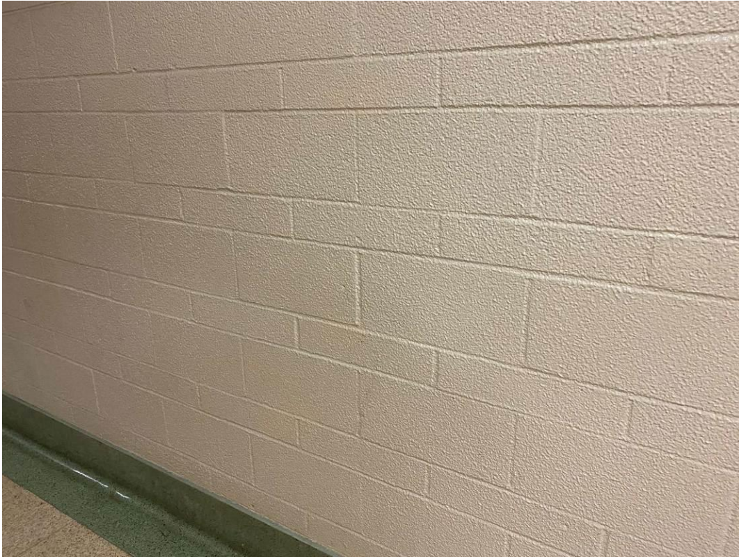
V0025 (None), Textured, Wall, Paint, Stairwell (Location #: 2990)
