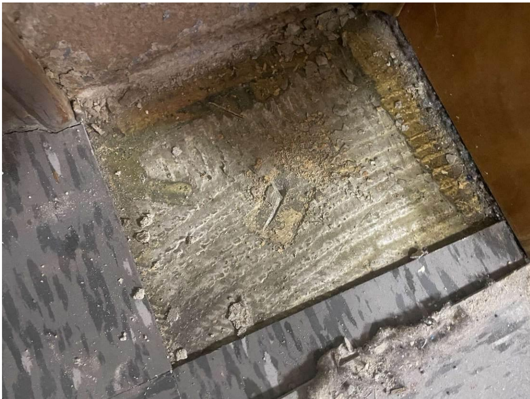
S0041A (None), Under Vinyl floor tiles, Floor, Floor Levelling Compound, Learning Commons (Location #: 2972)
