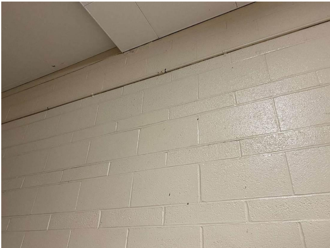
V0001(Lead, Low), Off white paint on masonry wall, Wall, Stairwell (Location #: 2990)
