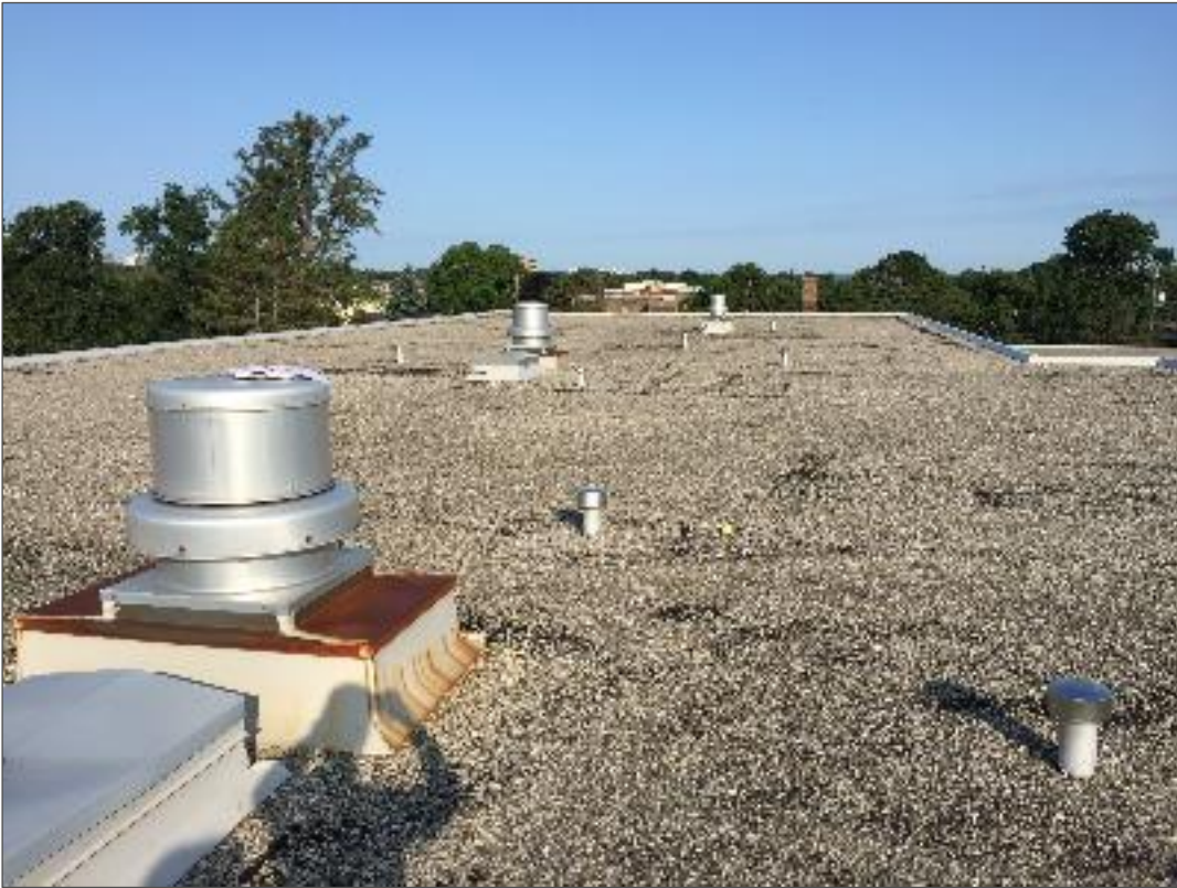
S0001A-C (None), Other, Roofing Materials, Roof / Exterior (Location #: 0) – (Photo from previous report)
