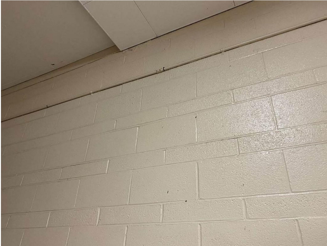
V0028 (None), Smooth, Wall, Paint, Stairwell (Location #: 2990)
