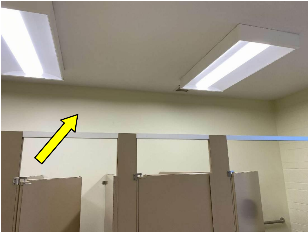
V0030 (None), Wall, Drywall and joint compound, Girls Washroom 2 (Location #: 2976)
