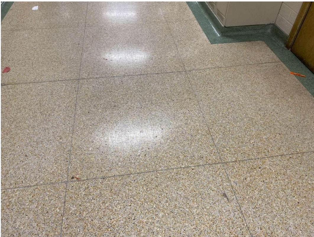
V0029 (None), Floor, Terrazzo, Corridor (Location #: 2984)
